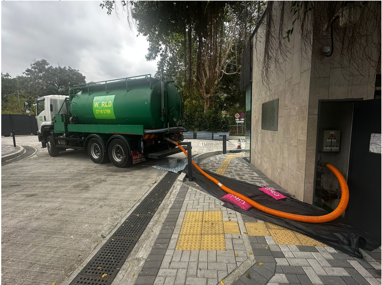
Figure 3.4 Photo Record - trucking away the wastewater of underground sewerage tank (human waste) –
