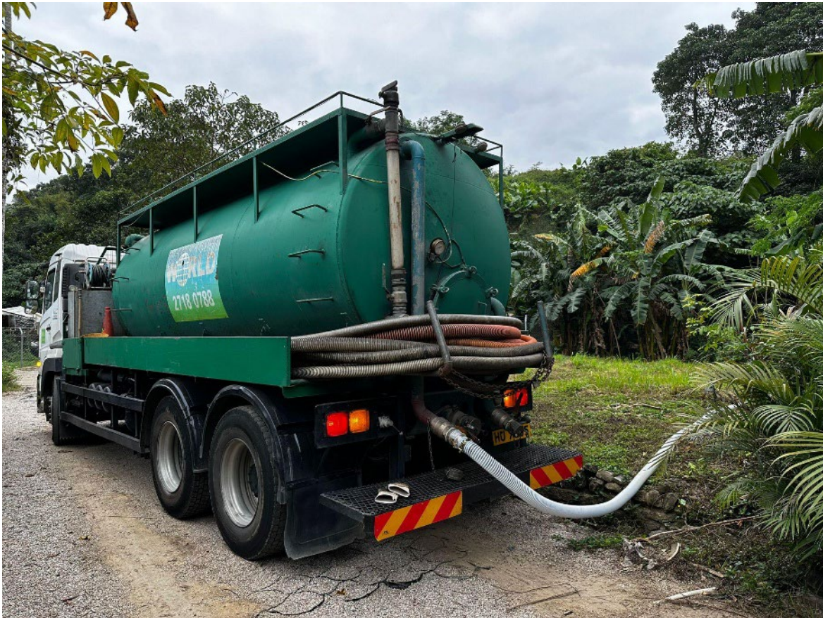
Figure 2.2 Photos of Vacuum Tanker trucking out the stormwaters
