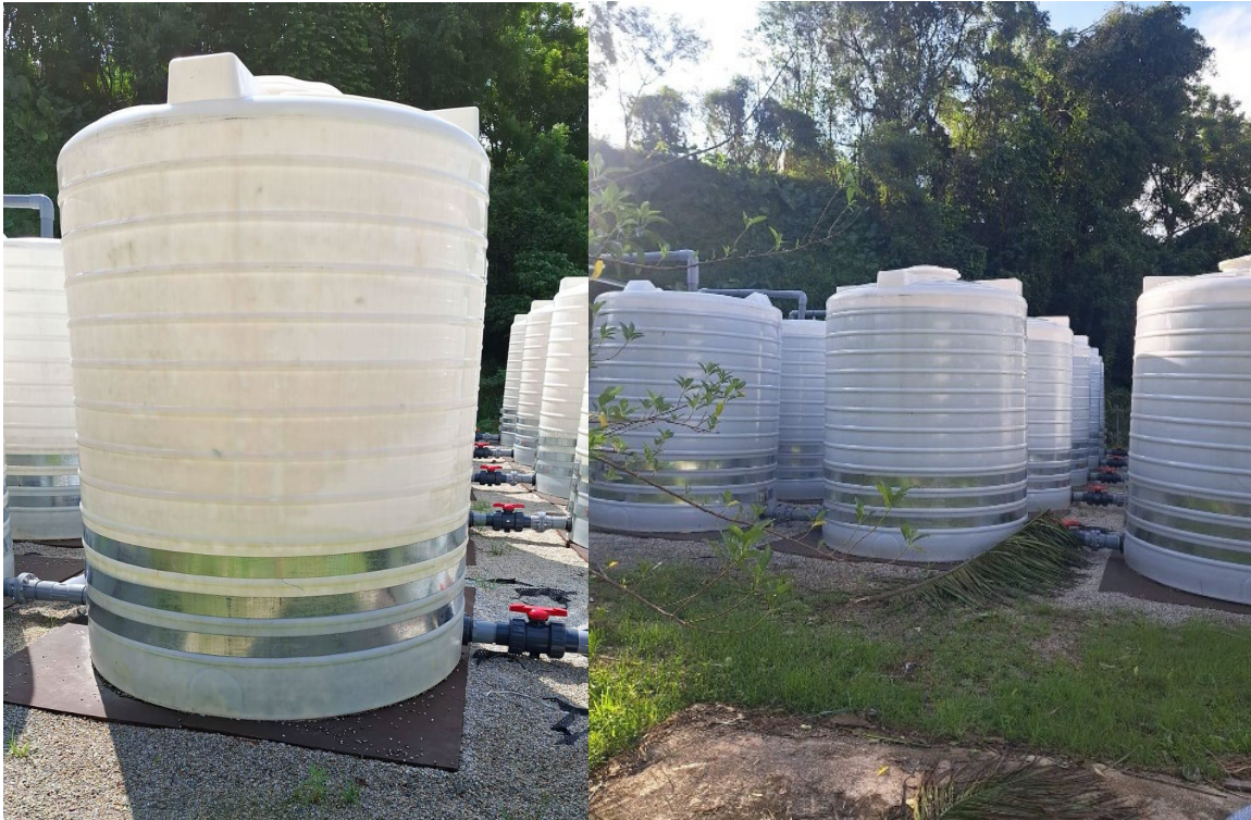
Figure 2.1 Photos records of temporary storage tankers for stormwater
